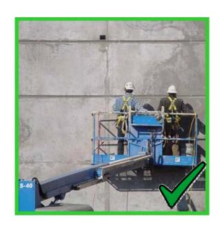
All pneumatic and hydraulic components must comply with ANSI A92.2.1969 and non-critical parts must have a burst factor of 2:1
